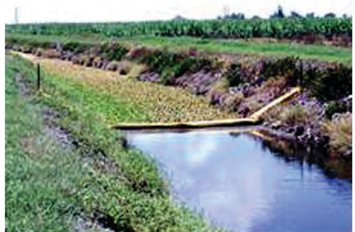
Figure 11. Weed booms (a) and trash racks (b) keep aquatic weeds from drainage pumps.
