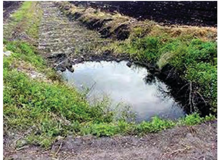
Figure 5. Typical field ditch sediment sump.
