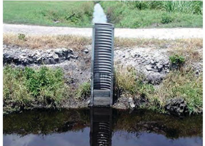
Figure 7. Riser boards slow drainage near pumps.
