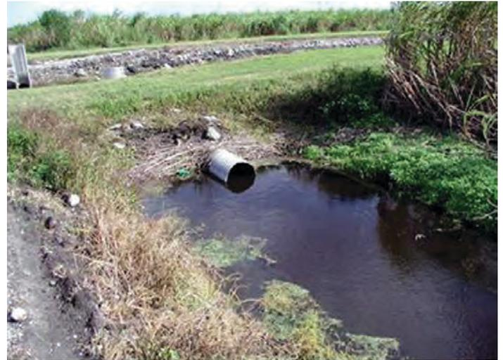
Figure 9. Raised culvert bottom reduces bedload sediment transport.
